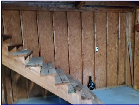
No railing on stairs, safety hazard
