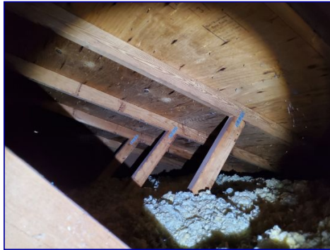
Possible moisture stains from previous roof leak
