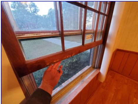
Window would not stay in up position.
