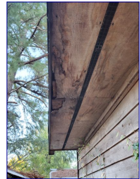
Delaminated soffit
