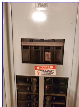
Bedroom 2 outer wall
