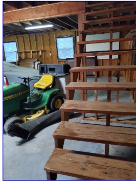
No railing on stairs, safety hazard
