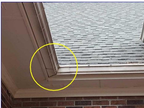
The gutters are dirty. Recommend cleaning the gutters to ensure proper water flow to the downspouts. Gutter leaks in this area.
